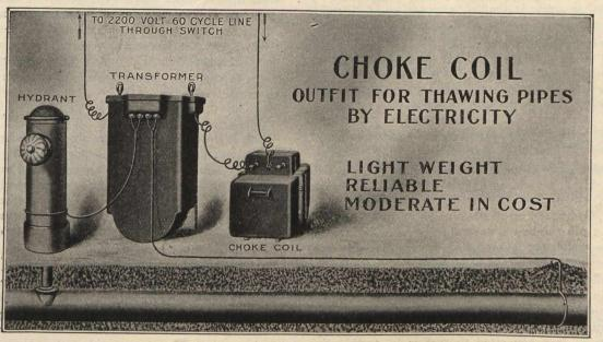
used in connection with the primaries of a standard transformer and one for lighter service, consisting of a transformer adapted for suitable secondary voltage adjustments, mounted in cast-iron top and bottom frames, and intended to be used directly on the primary mains The connections are simple and easily made, and the operator is entirely protected from injury.
