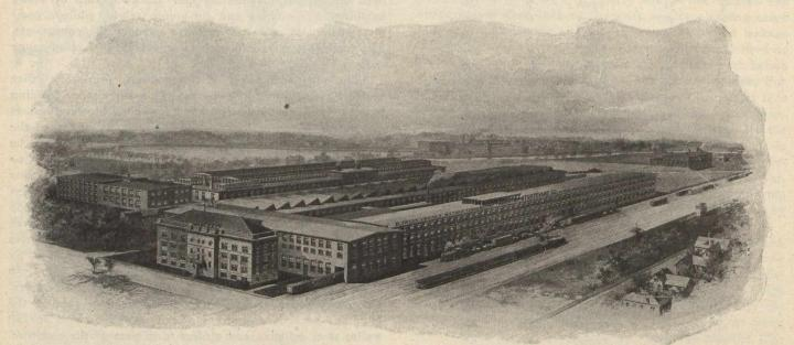
Fig. 8: Birds-eye View of B. F. Sturtevant Company's Works, Hyde Park, Mass., U.S.A. Machine Shop is the Central Building with Saw-tooth Roof.
