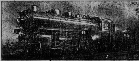
constructed under the direct supervision of Mr. W. H. Winterrowd, chief mechanical engineer of the C. P. R. The total weight of each engine and tender in working order is 480,000 lbs., the cytinders are 25 inches by 30 inches, the diameter of the driving wheels 76 inches, and the boller carries 300 lbs. steam pressuregives to the complex of the driving wheels 76 inches, and the boller carries 300 lbs. steam pressuregives to 42,000 lbs.
