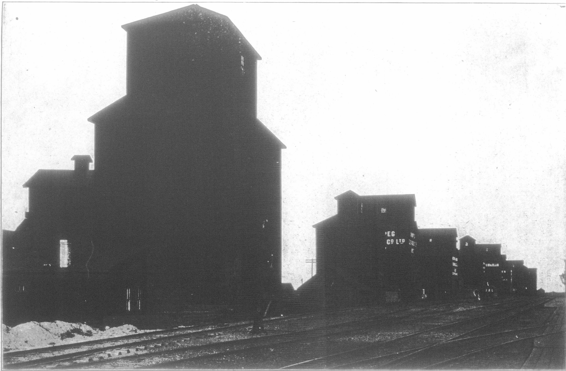
Elevators in Irrigated District which guarantees big crops.
