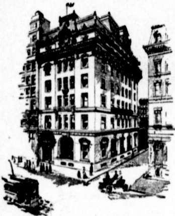
CANADIAN BRANCH LONDON & LANCASHIRE LIFE HEAD OFFICE BUILDING, MONTREAL HAL BROWN, GENERAL MANAGER.
