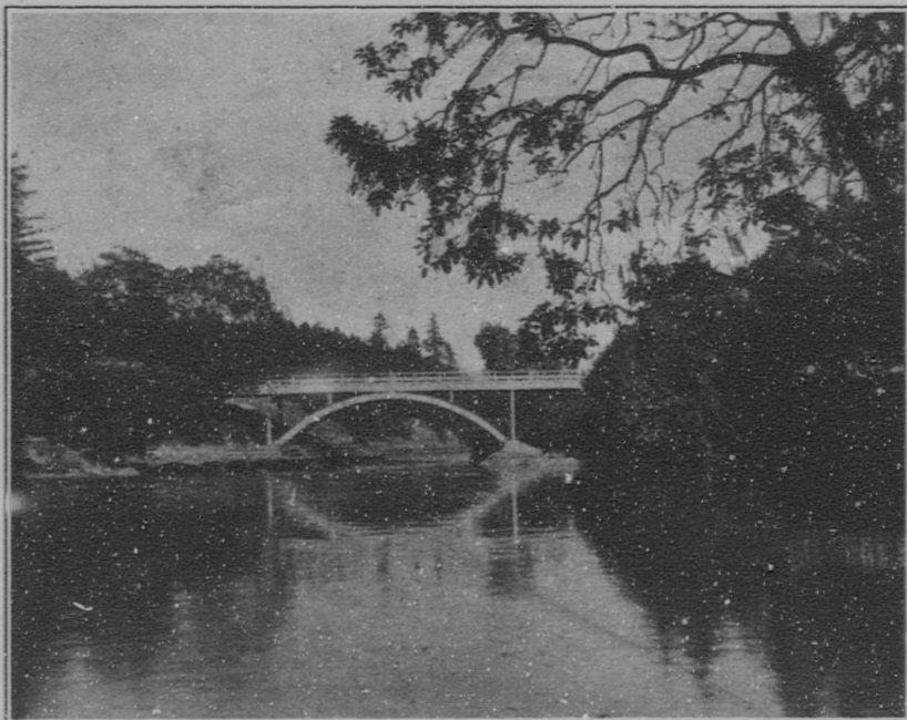
The Gorge Bridge, Looking Towards the B.C.E.R. Park
