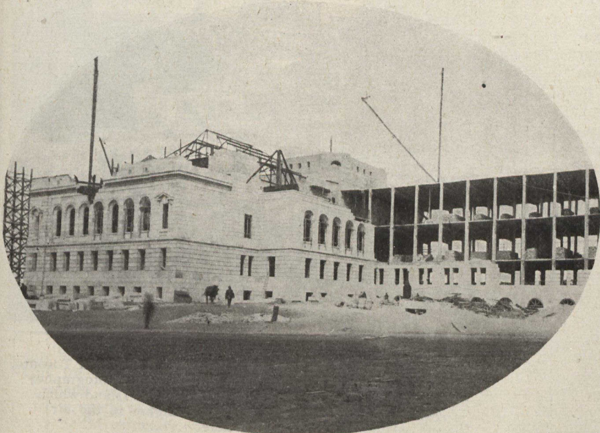
The Capitol of Saskatchewan, now Building at Regina.
