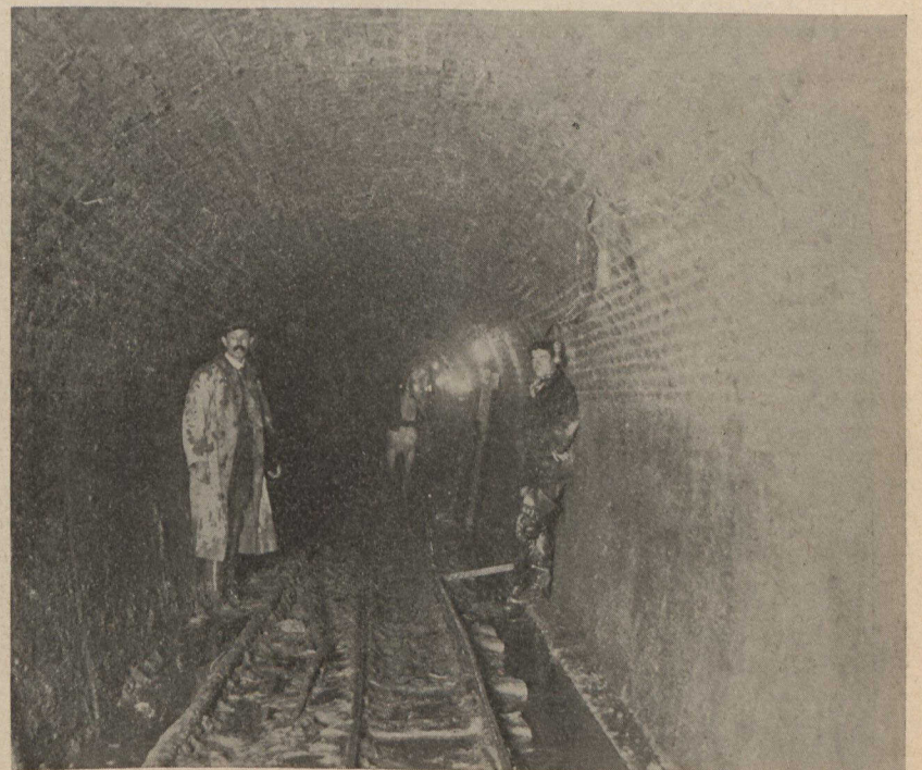
Where Water will Soon be Pouring Through
