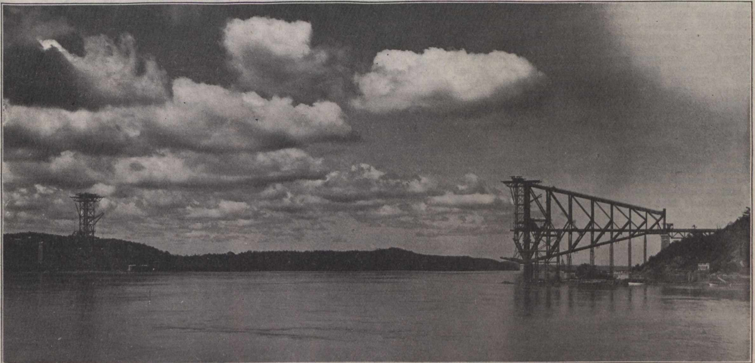
The Quebec Bridge, showing Progress of Construction to June 18.
