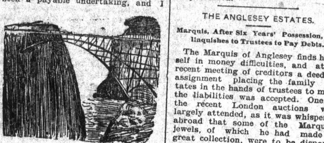
BRIDGE OVER ZAMBESI GORGE.
