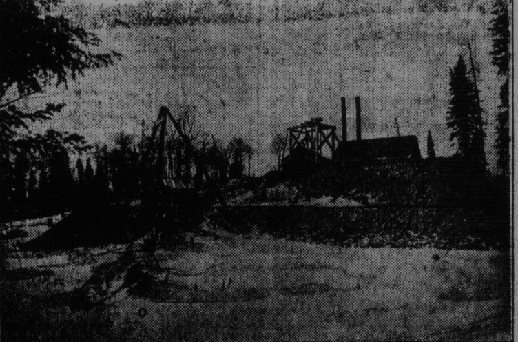
Buildings of the Foley-O'Brien mine at Porcupine, which were burned in last week's fire.
