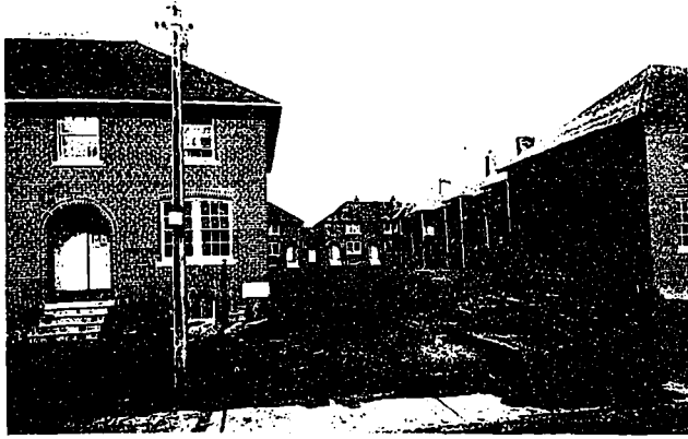
VIEW OF SPRUCE COURT, TORONTO.
