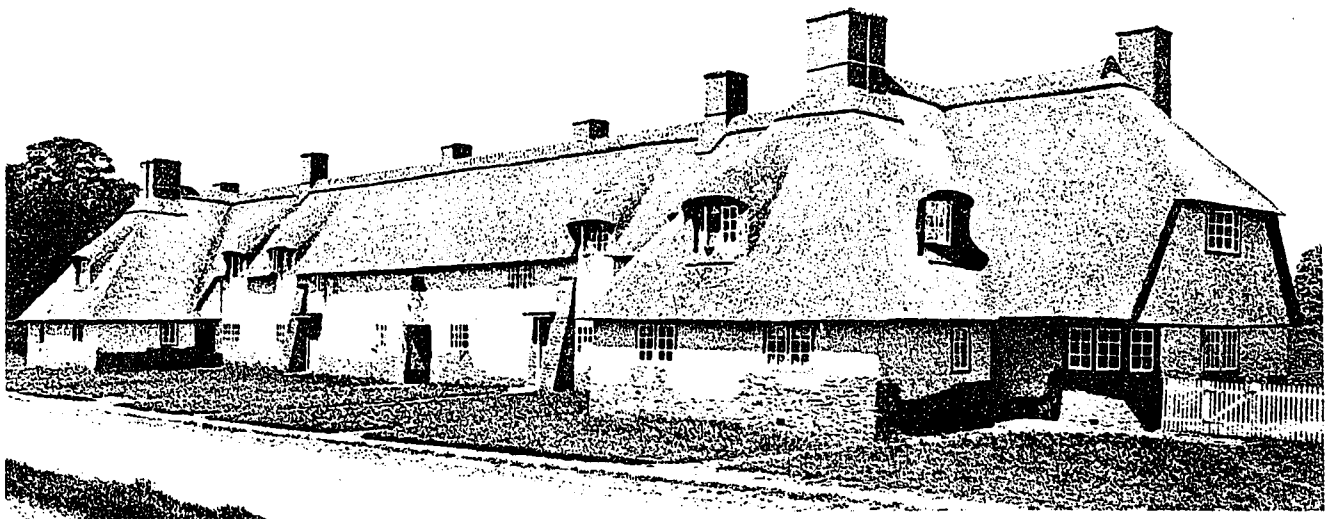
COTTAGES NEAR RUGBY, ENGLAND, BY E. L. LUTYENS, ARCHITECT.
