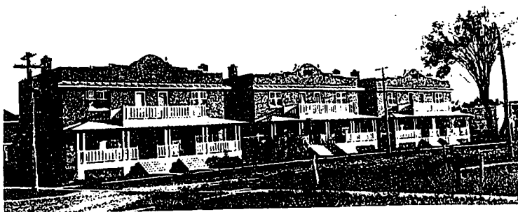
NO. 1.—SEMI-DETACHED HOUSES AT ST. LAMBERT.
