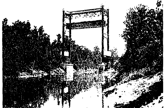
BRIDGE AT BIG CHOCTAW BAYOU, LOUISIANA.
