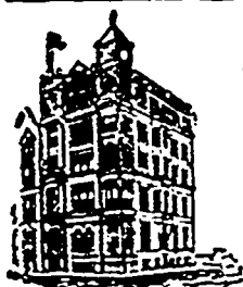
HEAD OFFICE BUILDING, MONTREAL
