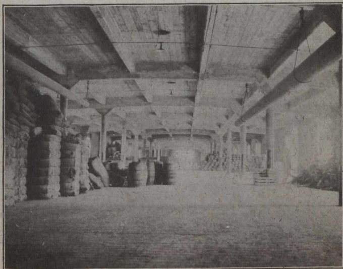
Fig. No. 5—Furness Withy Pier—Interior of Shed
