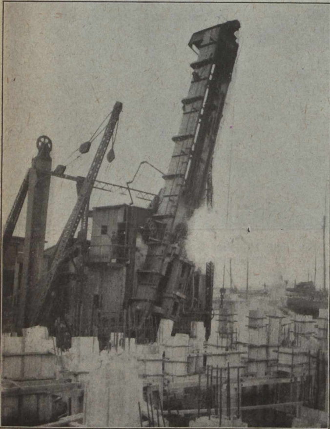
Fig. No. 11—Pier No. 2—Driving Batter Pile
