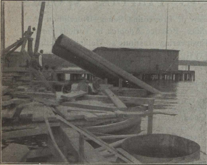
Fig. No. 3—Furness Withy Pier—Tipping Steel Cylinder into Water
