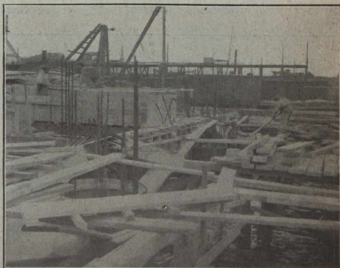
Fig. No. 6—Furness Withy Pier—Bent of Cylinders Filled and Braces Set
