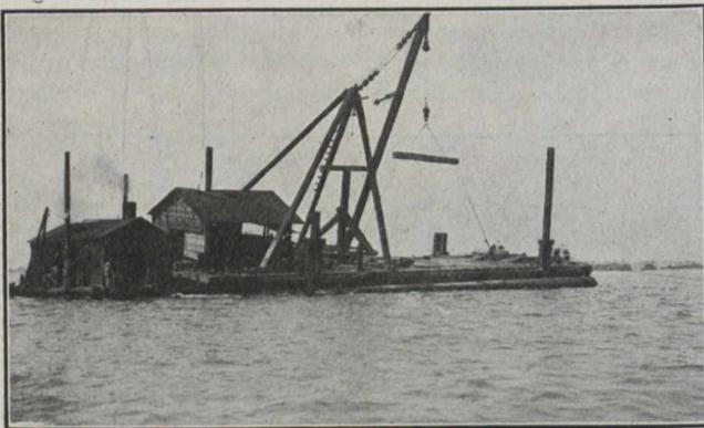
Outfall Sewer, Lowering a 100-ft. Section of the 60-in Steel Pipe.
