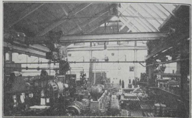
Lifting Block and Overhead Crane.
