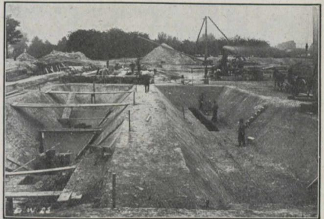
Sedimentation Tanks, Showing Excavation and Bottoms.
