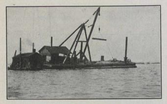
Outfall Sewer, Lowering a 100-ft. Section of the 60-in Steel Pipe.
