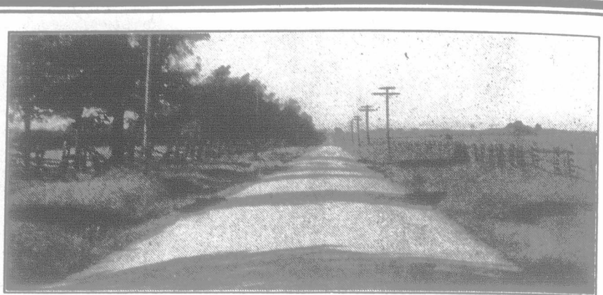
Kennedy Roads, Scarboro Township, York County Highway Board, Ontario. Treated with "Tarvia-B" in 1915.
