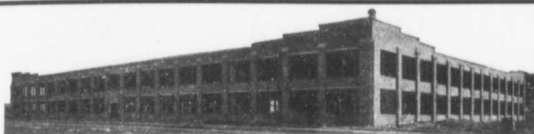
Portion of Plant of A. J. King Piano Co., Bluffton, Ind. Built with Ideal Concrete Machinery.
