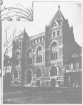
ST. PAUL'S PARISH HALL.
