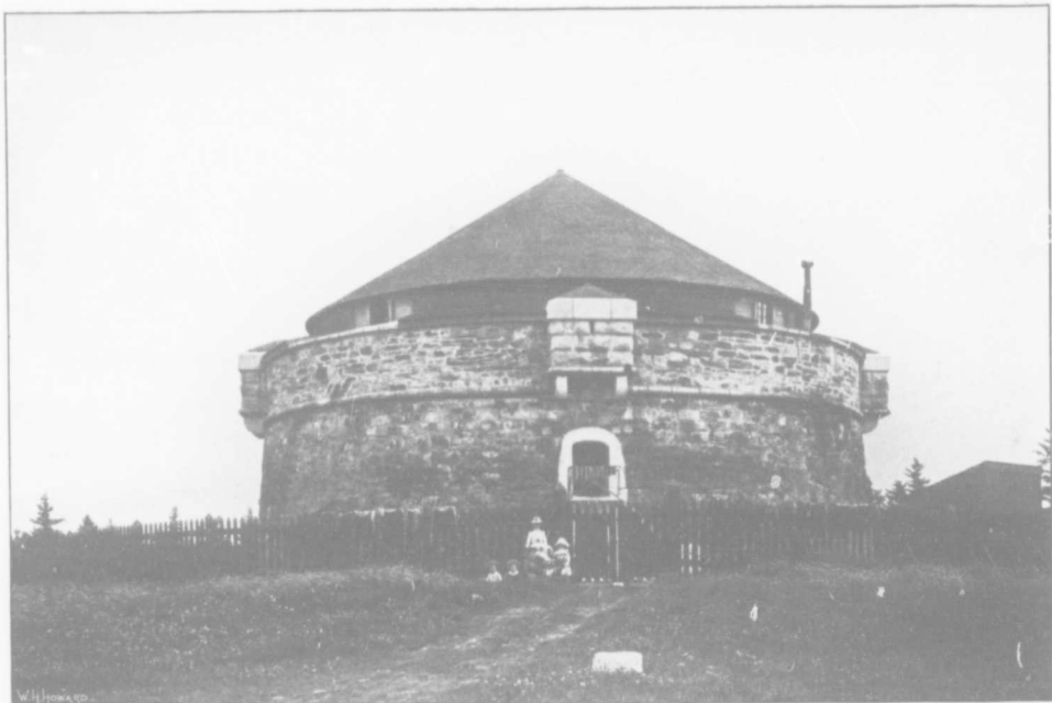
OLD MARTELLO TOWER, POINT PLEASANT PARK
