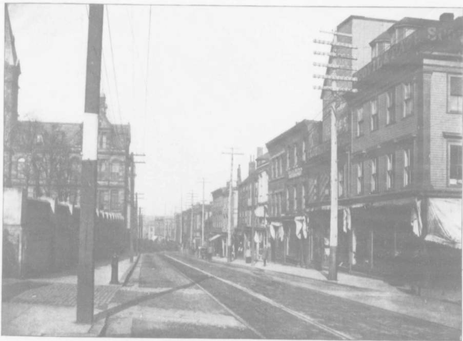
BARRINGTON STREET, LOOKING NORTH FROM GEORGE STREET.
