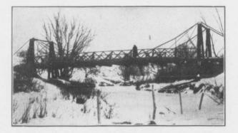
attached to concrete anchorages deeply embedded in the earth banks, and all the underground parts are protected by concrete. The cables are 13%-inch crucible caststeel, galvanized, with steel centres. They are composed of seven strands of seven wires each. They were manufactured especially for suspension bridges by the Roeblings, Trenton, N.J.
