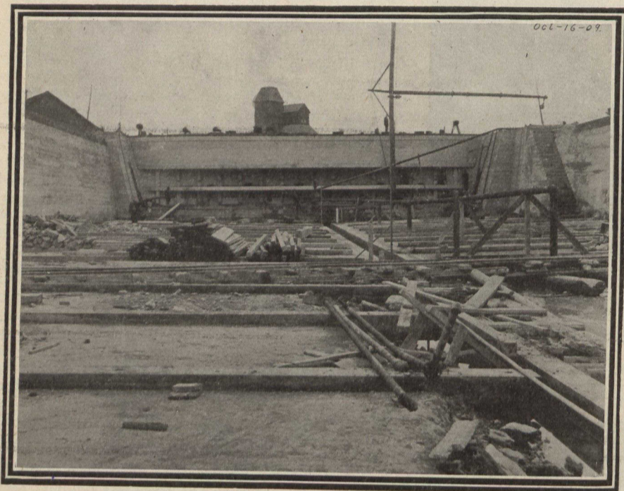
The new Dry Dock at Collingwood, from a photograph taken before completion, showing the pontoon gate. October 16th, 1909.
