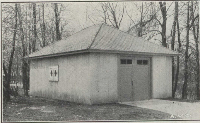
Garage at Woodlands, P.Q., Owned by Mr. W. G. Ross, Pres. of Harbor Commission, Montreal. Roof of Asbestoslate—Walls of Asbestos Corrugated Sheathing.
