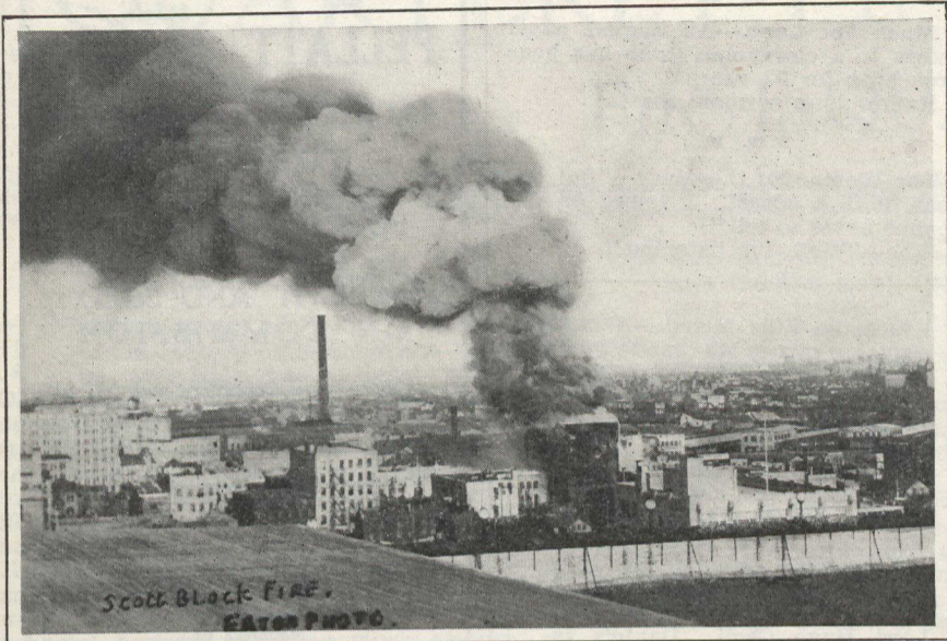
A graphic picture of the Scott Block fire in Winnipeg, on March 23rd. This fire cost $250,000, and might have been much more serious but for an excellent fire-fighting service.
