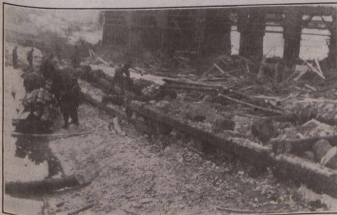
Fig. 7.—The First Cofferdam Being Removed
