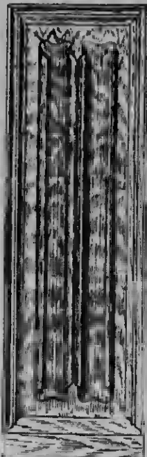
Fig. 1844.—Framed Panelling in Lower Portion of Pulpit.
