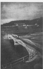
ROMAINE'S BRIDGE. This is the first reinforced concrete bridge built in the country and all parts, even the rails, are of concrete.
