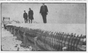
FLUME OF ELECTRIC PLANT AT PORT UNION-FIRST STAVE FLUME CON-STRUCTED IN NEWFOUNDLAND.
