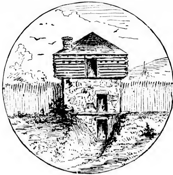
Block House. Built in 1780.
