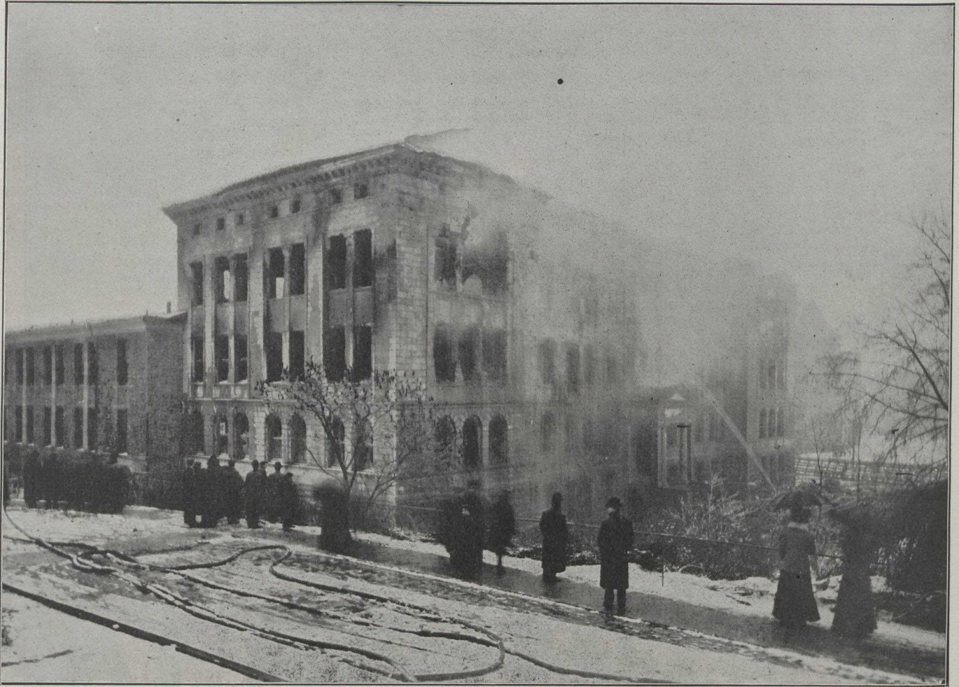
The Fires at McGill Fire on Friday morning, April 5th, utterly destroyed the Macdonald Engineering Building, one of the finest of the handsome group on the Campus. Its equipment was second to none on the continent. The origin of the fire is a mystery. This picture shows the building through a veil of steam and smoke.
