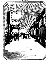
DELCO-LIGHT IN THE RAILWAY STATION
