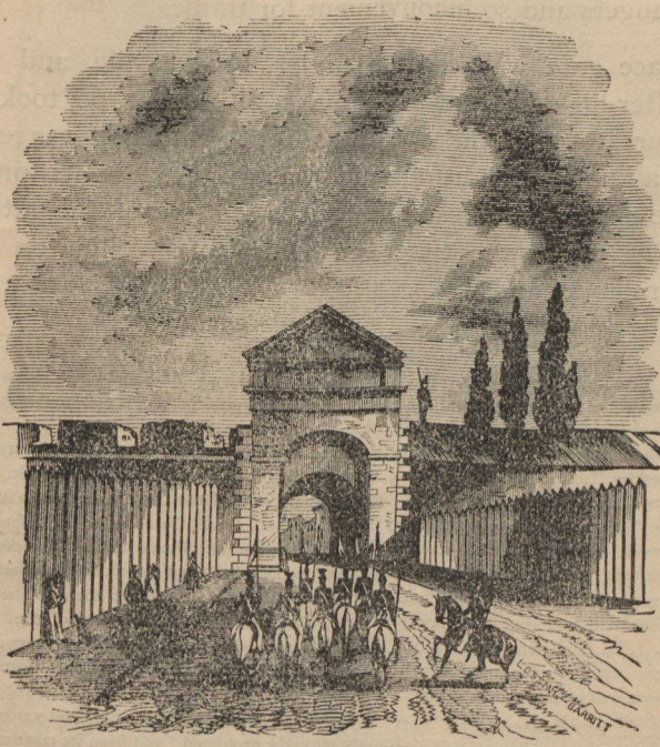
ST. LOUIS GATE, DEMOLISHED, AUGUST, 1871.
