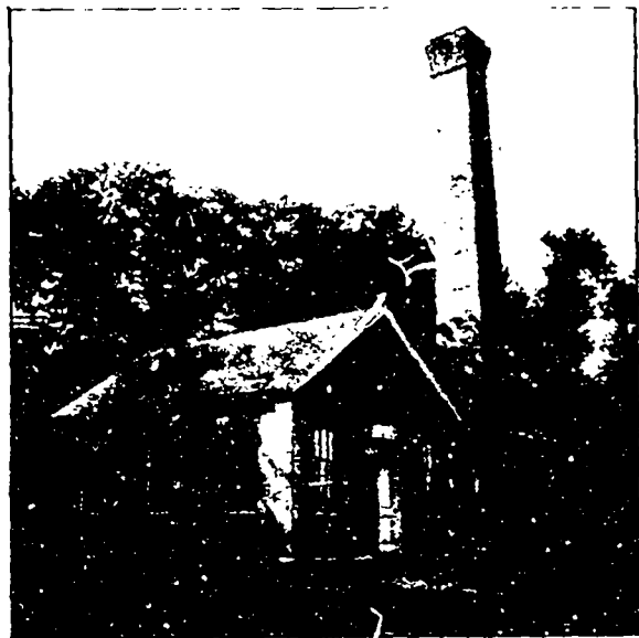
PUMPING STATION, STELLARTON, N.S.
