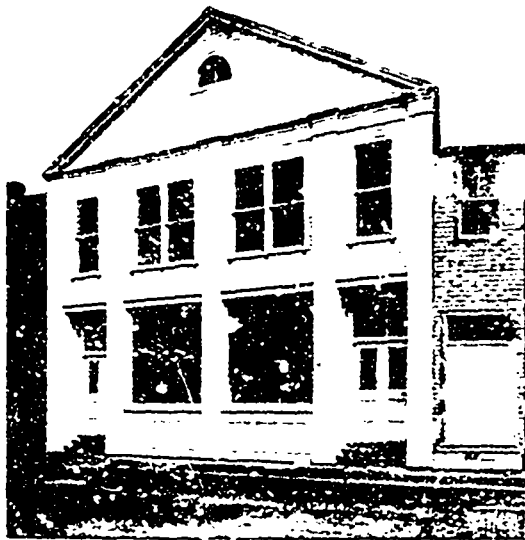
THE PICTOU ADVOCATE BUILDING, IN COURSE OF CONSTRUCTION, PICTOU, N.S.
