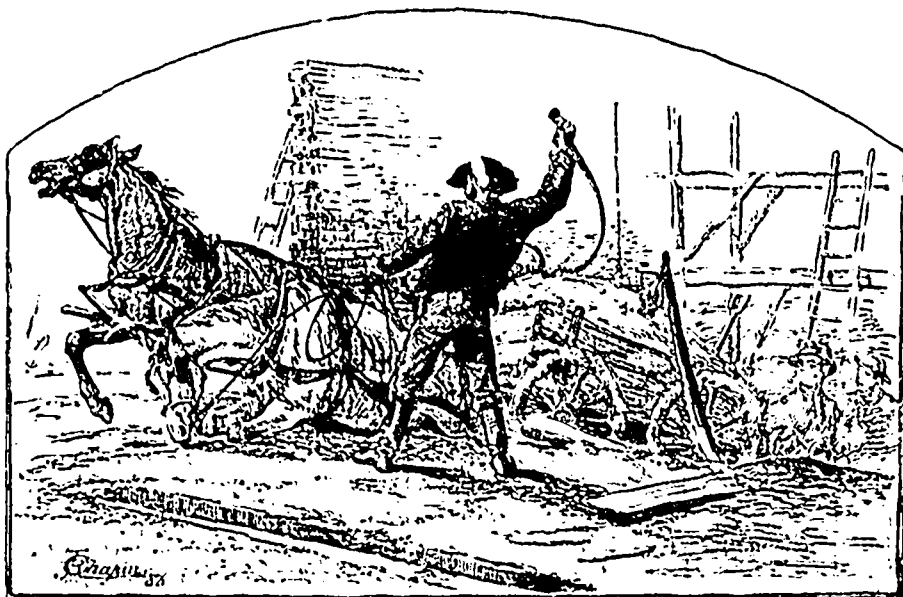
BROKEN DOWN BY OVERLOADING.
