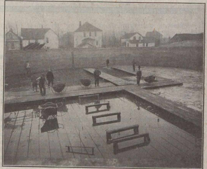
POURING FLOOR FOR RESERVOIR
