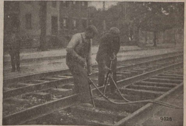
TWO-TOOL TIE-TAMPING OUTFIT SHOWS 38% SAVING IN COST OF WORK
