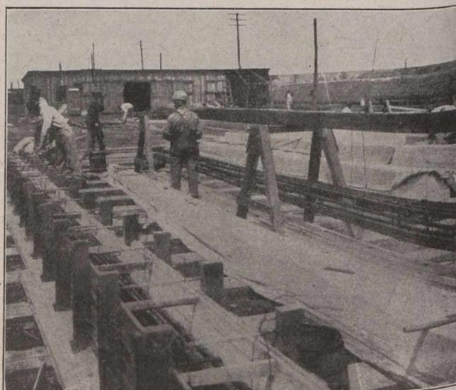
Manufacture of Concrete Telegraph Poles, Showing Skeleton Frame Suspended in Place; Frame in Form, Ready for Pouring, and Finished Pole.
