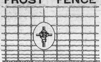
This fence is made in Canada enitrely of Canadian products. All the wires are full size true to gauge. Laterals and uprights are all No. 9 Hard Steel, well galvanized stock. Laterals are given a deep and continuous wave for "give and take." These coils or waves serve like a spring seeping the fence tight throughout all seasons and under all conditions. It used by the principal farmers everywhere. The cost to you is no more than the price of other fence of equal weight. Insist on getting it.
