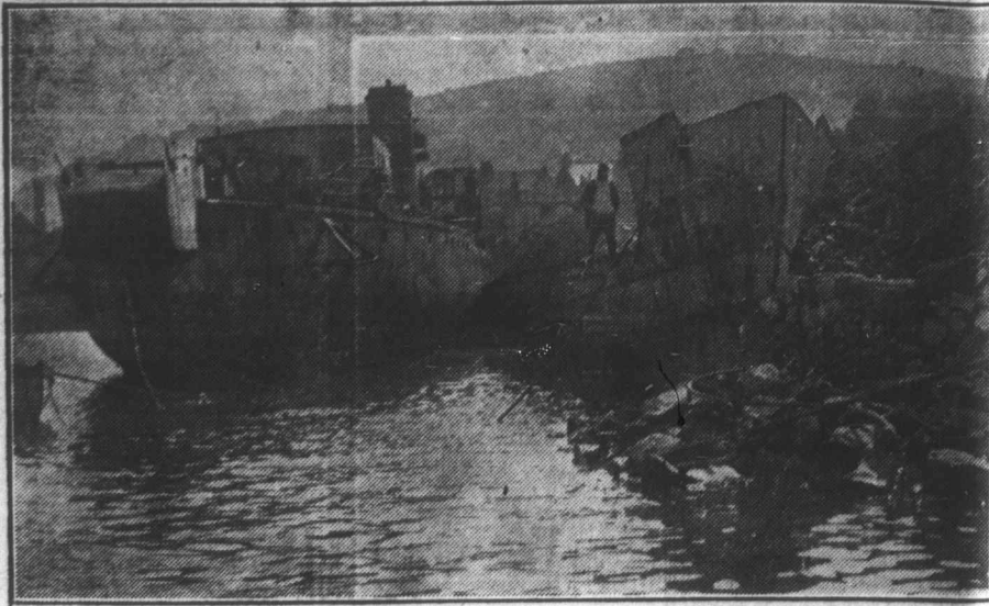
SEA WALL OF OBSOLETE WARSHIPS
