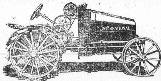
8-16 International—Valve in head Motor, THROTTLE GOVERNOR regulates fuel to load, friction Clutch Pulley.
