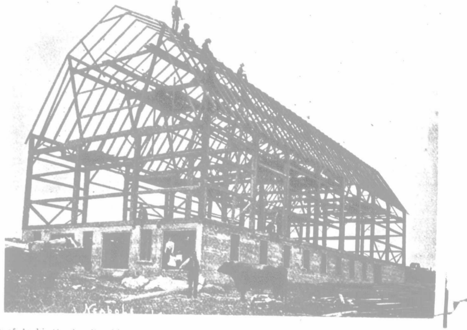
Barn of Archie Crozier, Beaufort, Ont. Size of wall, 15 x 120 ft. Wall, cistern and floor built with THOROLD CEMENT. The holes showing along the top of the wall are for ventilation.
