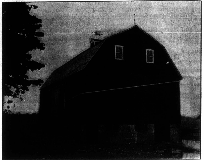
BARN OF WM. PATTON, SOUTH CAYUGA, ONT. Size of Basement Walls, 36 x 60 x 9 feet. Built with Thorold Cement.
