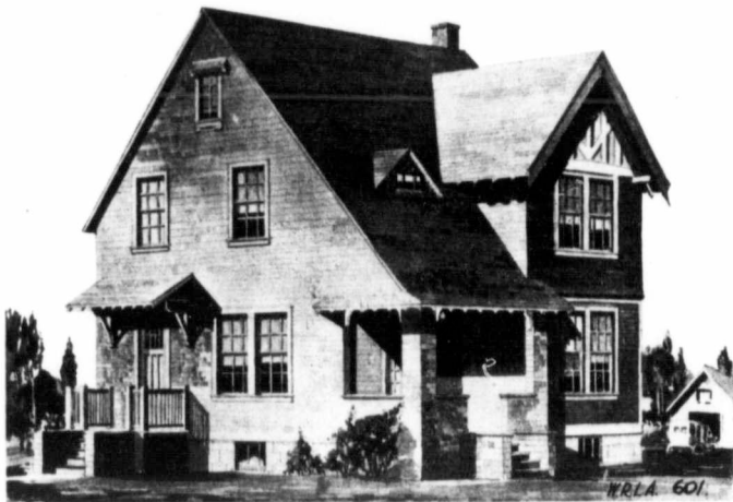
A pleasing modern adaptation of an Old English design, with Duplex air-space wall construction shown on working drawings. Built according to construction specifications, you will have a life-long home of comfort.
