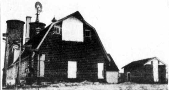
Dairy Barn, Silos and Milk House Built of Hollow Tile
