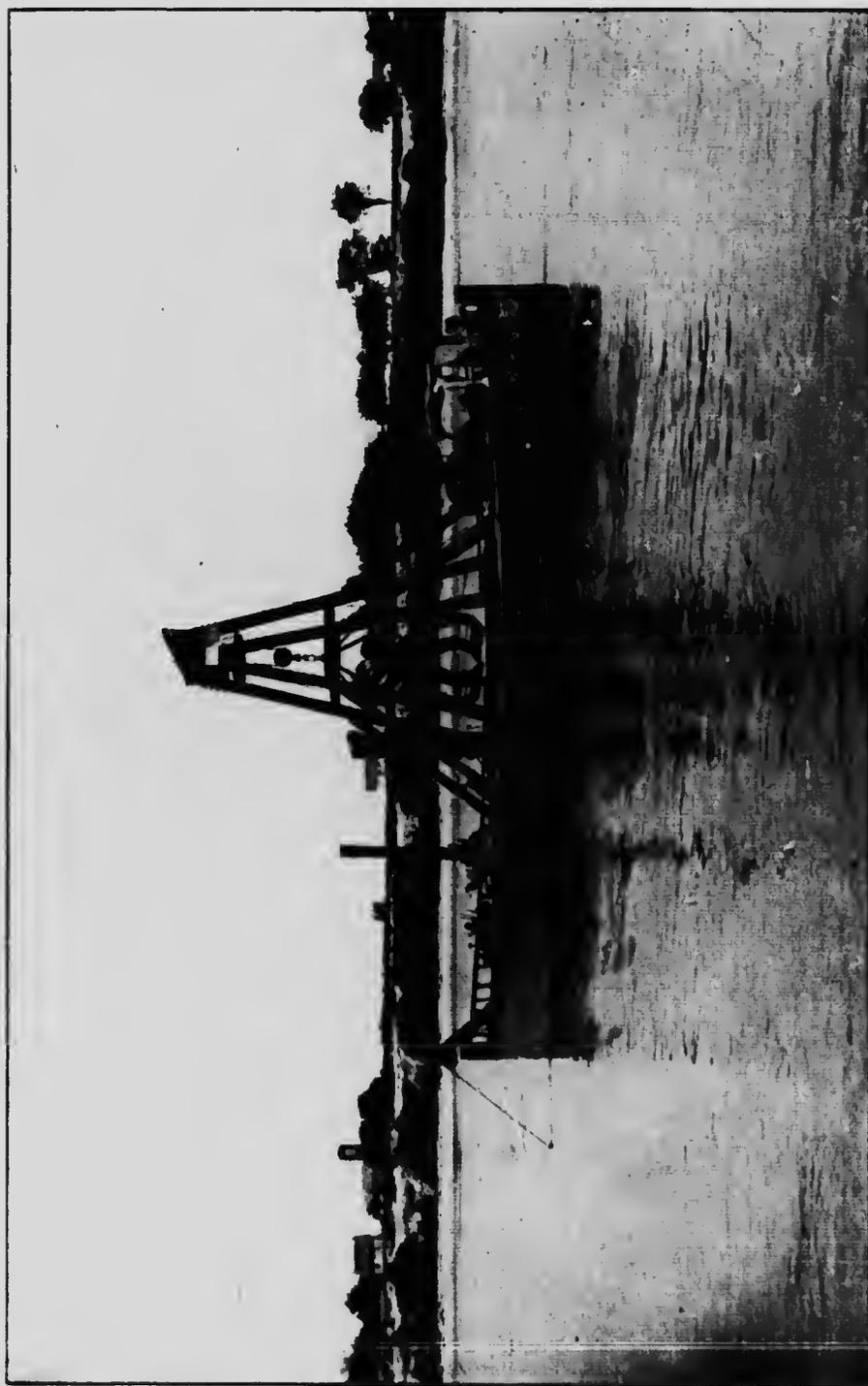
STONE LIFTER NO. 3, SHOWING GRIPS CAPABLE OF LIFTING BOULDER WEIGHING 30 TONS.
