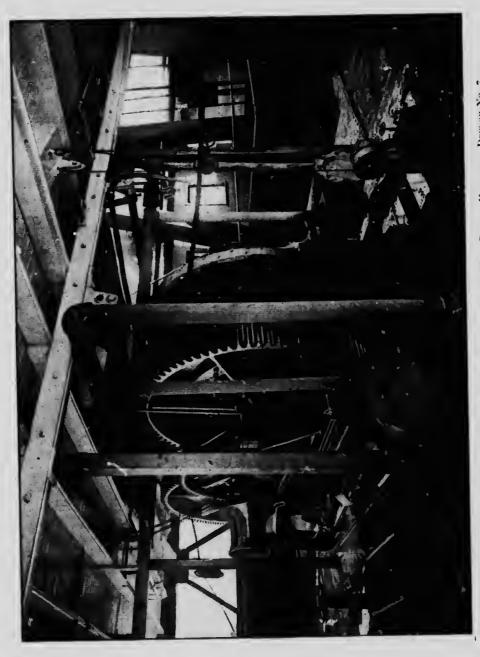
DOUBLE BOW-BREASTING WINCH ON MAIN DECK, UNING STEEL WIRE CABLES, HYDRAULIC DREIGH NO. 7.
