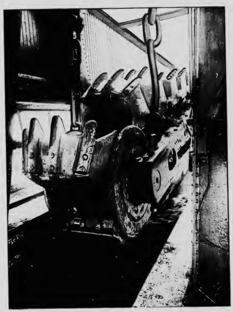
Elevator Duedge, shoaing Cast Steel Buckets for Work in Soft Rock, Lover Tumbler and Connections.
