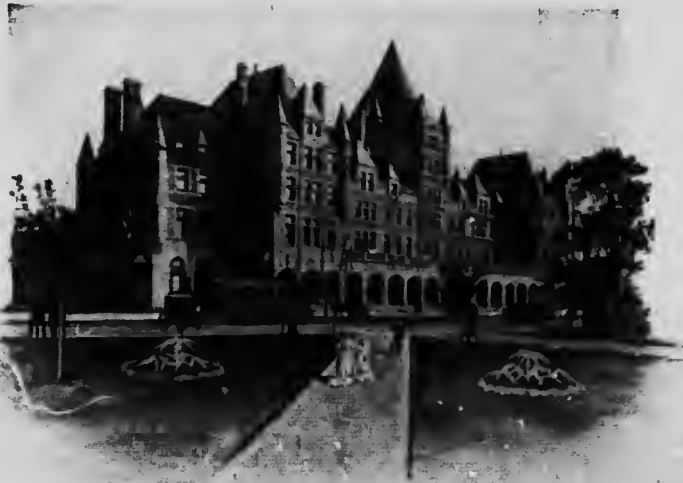
Place Viger Hotel and Passenger Station, Montreal.
