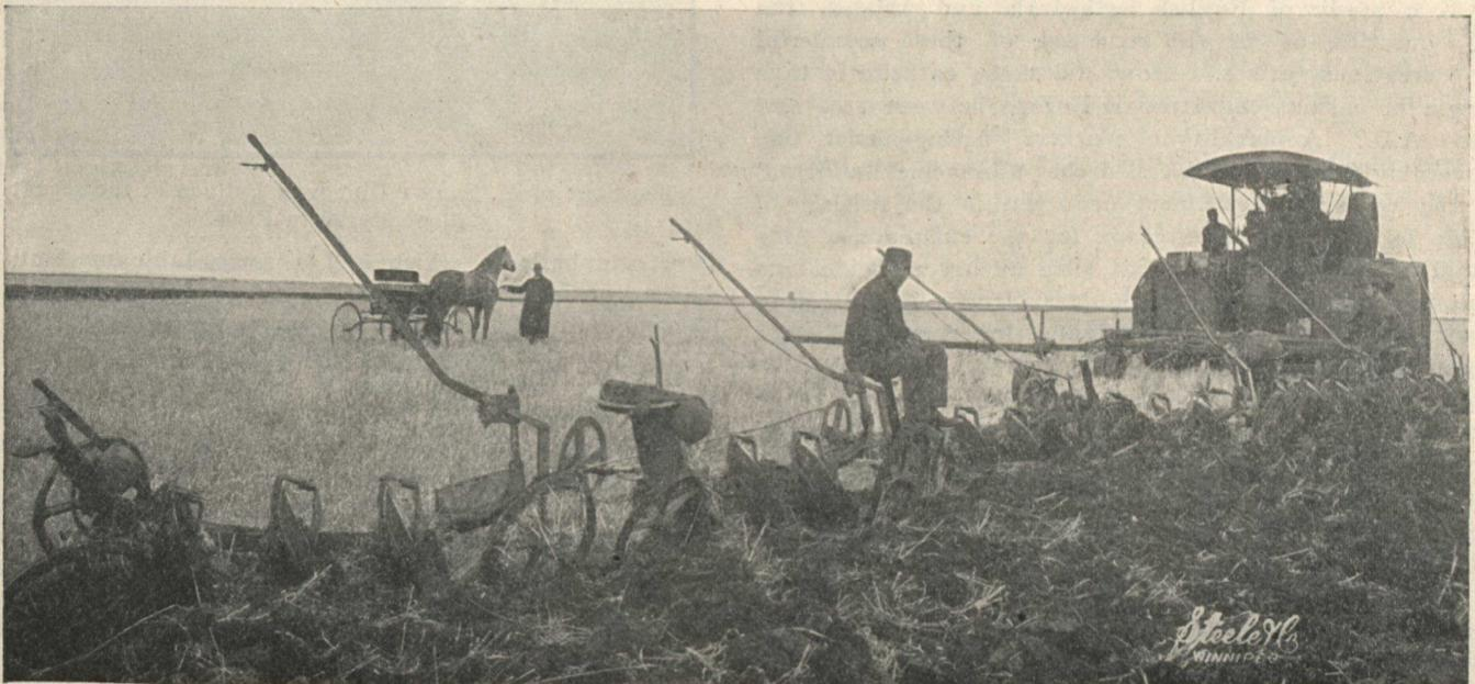
In the West Steam Ploughs are used for Breaking.
