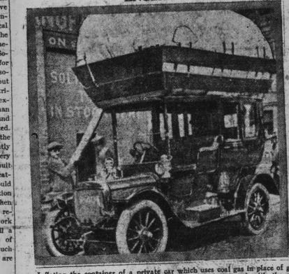
Inflating the container of a private car which uses coal gas in place of gasoline. The pipe shown conveys gas from a standard connection with the main to the flexible balloon into which it is just as if passing to an ordinary tank.
