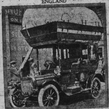
Inflating the container of a private car which uses coal gas in place of gas The establishment of one would make for better civic government as well as
