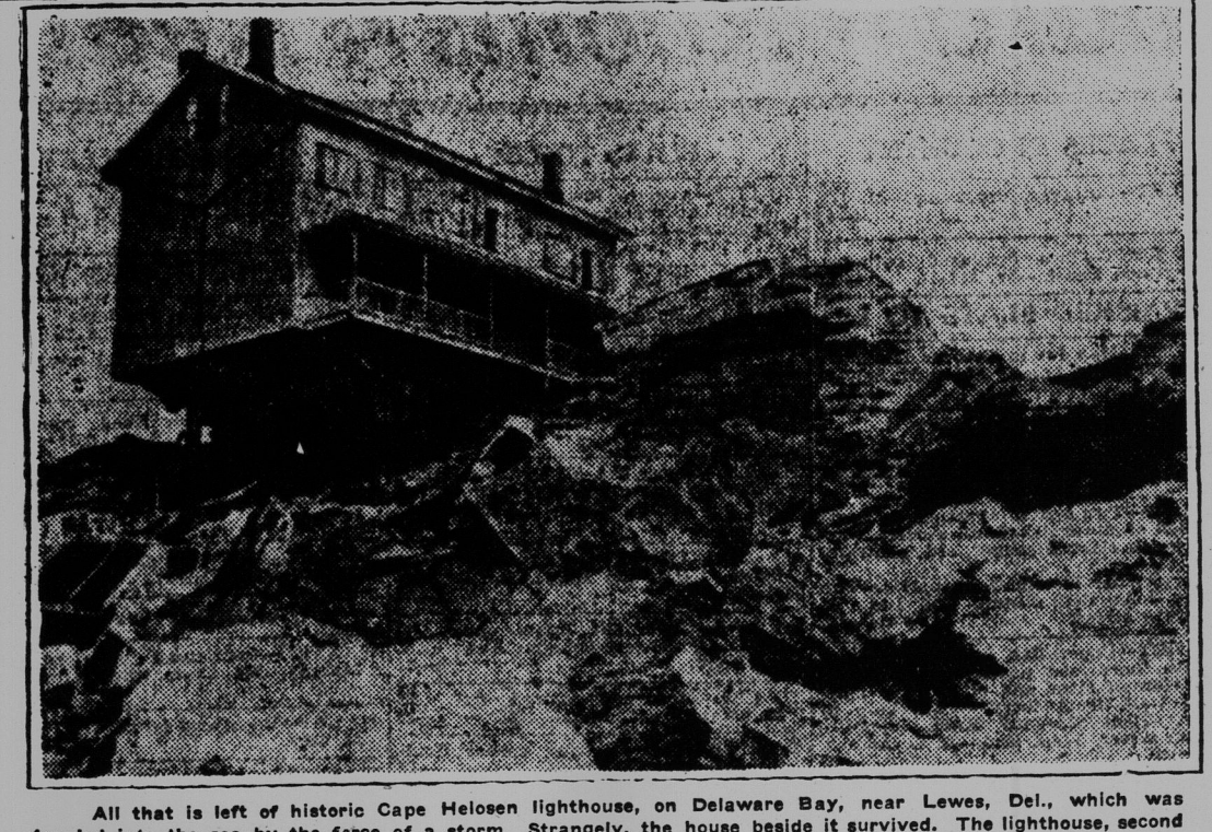
All that is left of historic Cape Helson lighthouse, on Delaware Bay, near Lewis, Del., which was toppled into the sea by the force of a storm. Strangely, the house beside it survived. The lighthouse, second oldest on the Atlantic coast, was constructed by the British in 1755.
