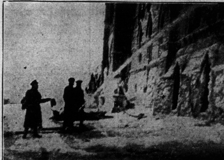
Tons of water were thrown into the burning building, which soon became coated with ice. This picture was taken at 8 o'clock Friday morning.
