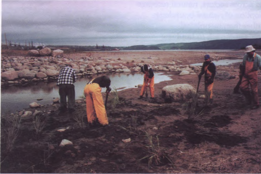
Rehabilitation of a bulrush marsh at the outlet of the Ha Ha! River in Quebec. This project was initiated as a result of the Saguenay River flood in 1996. Photo credit: Ghislain Sylvain.
