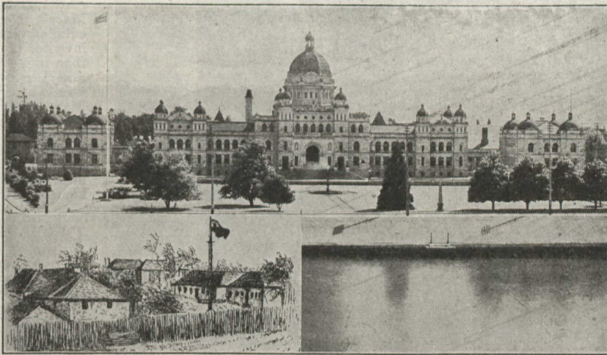
The old and the new: showing the British Columbian Legislative Buildings at Victoria from the waterfront, and inset at the bottom, a view of Fort Victoria, half a century ago.
