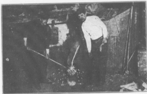
Wrong way to catch iron. Cutting the stream away from the furnace.
