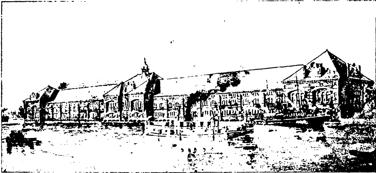
Power House, American Side.
